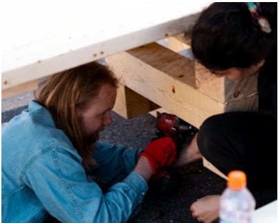
Building a community table
